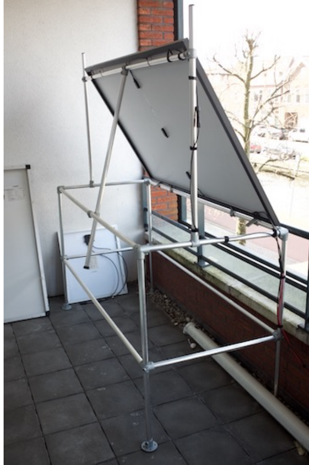
Figure 2.2: Solar panel used by Louwrentius with a rated power of 370 W [4].
